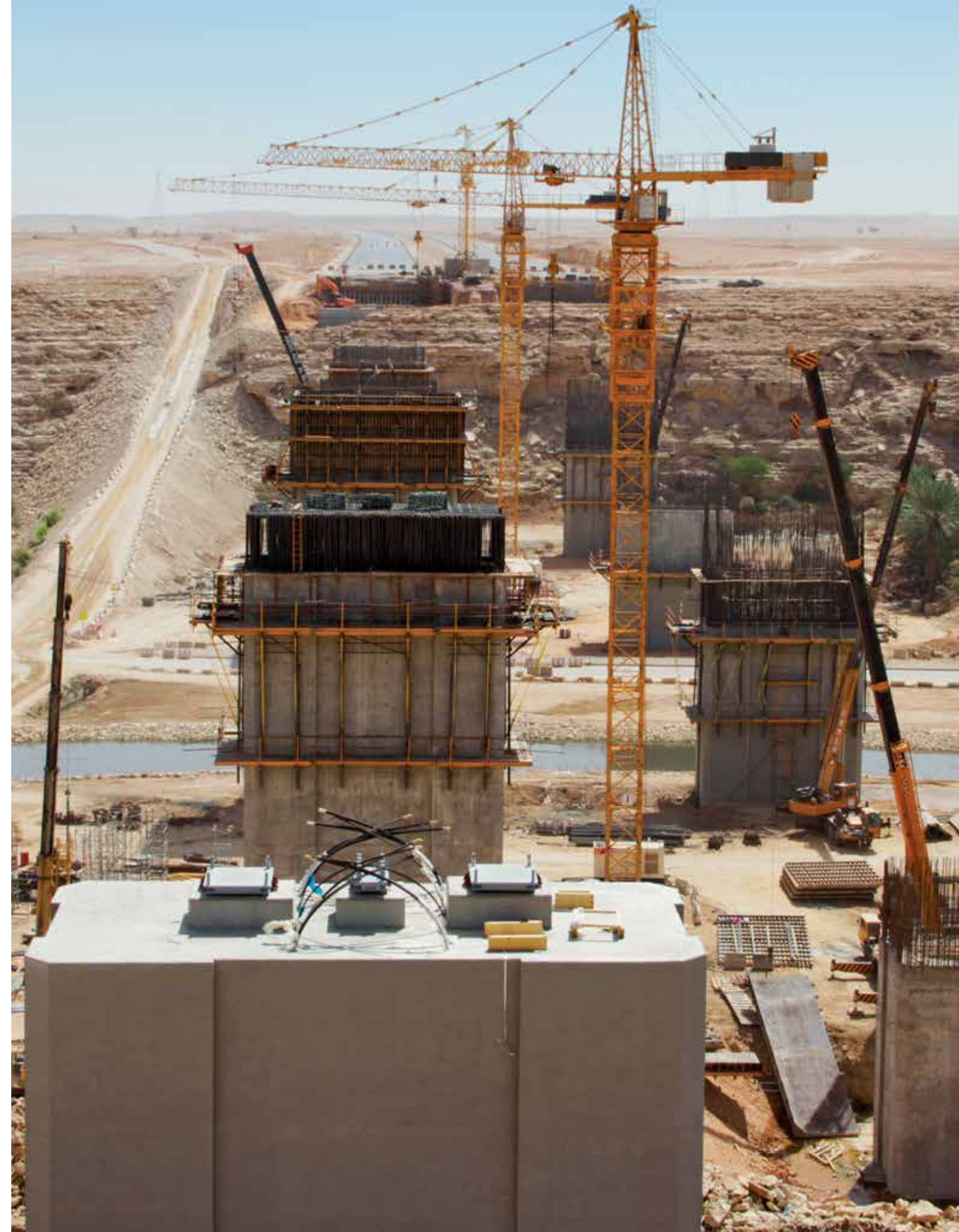
Wadi Hanifa Viaduct, Riyadh (Saudi Arabia)
