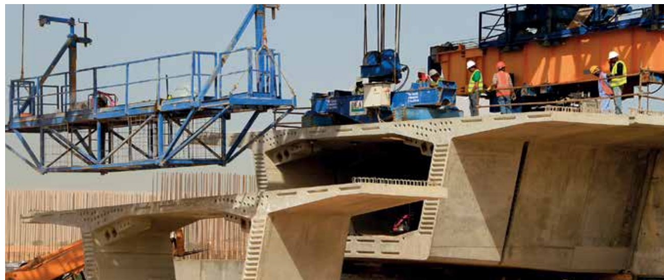
Wadi Hanifa Viaduct, Riyadh (Saudi Arabia)
